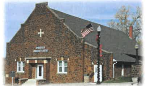
Springfield Community Building
